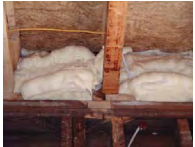
EA55 Spray Foam Insulation at Rim Joists
