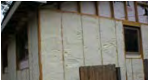
Spray foamed exterior curtain wall
