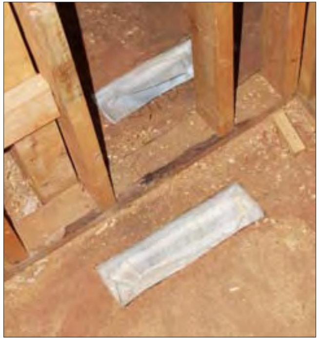
EA71 Duct Protection During Renovation
