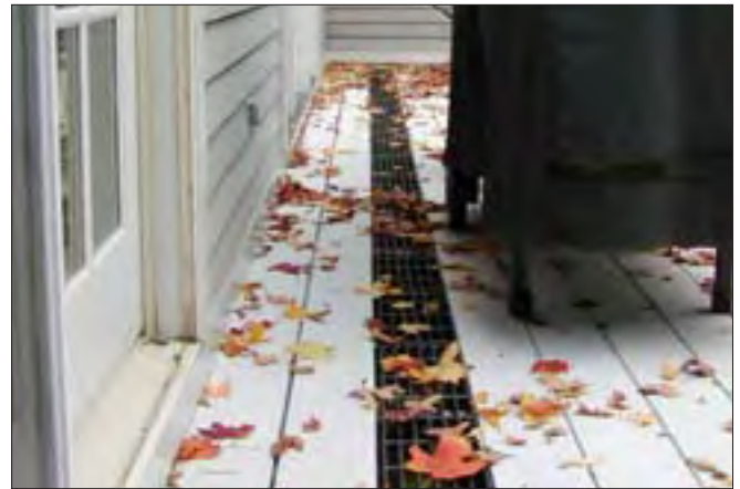
IDP25 Drip-Through Deck Grating on Gutterless Eaves
