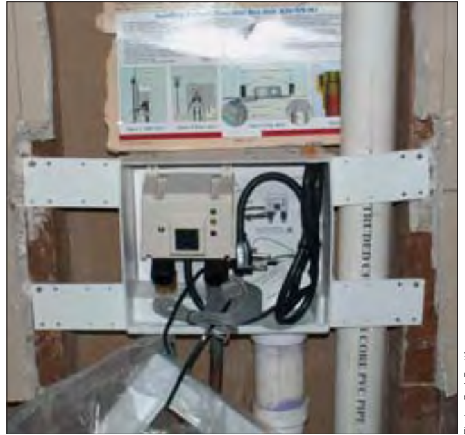
MR125 Alternative to Drain and Pan: Electronic Leak Detection for Clothes Washer
