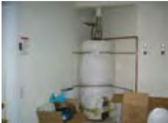
Before – low-efficiency, natural draft water heater
