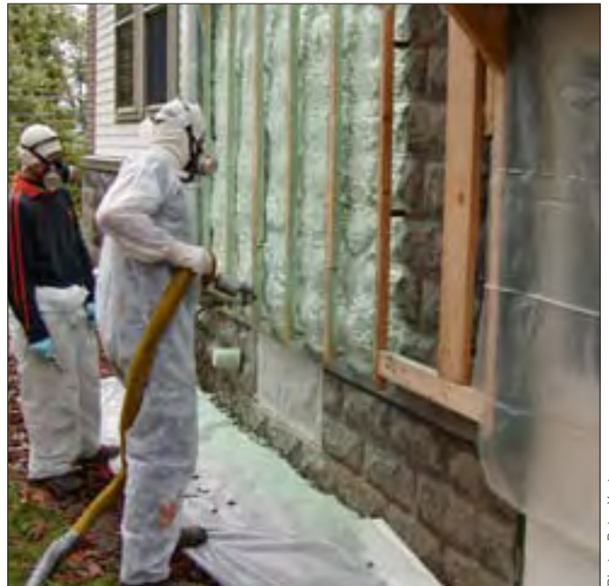
EA45 Exterior Wall Spray Foam Insulation
