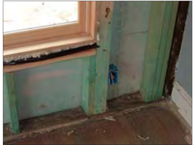
IDP23 Borate Insect Treatment of Framing
