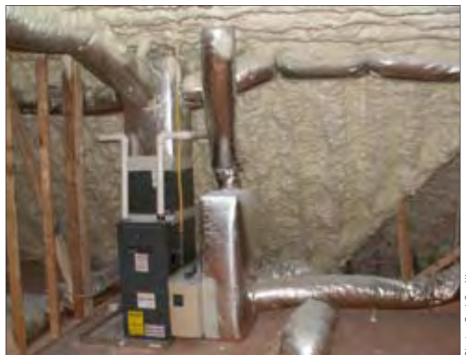
EA49 Spray Foam Insulation at Roof Line for Conditioned Attic
