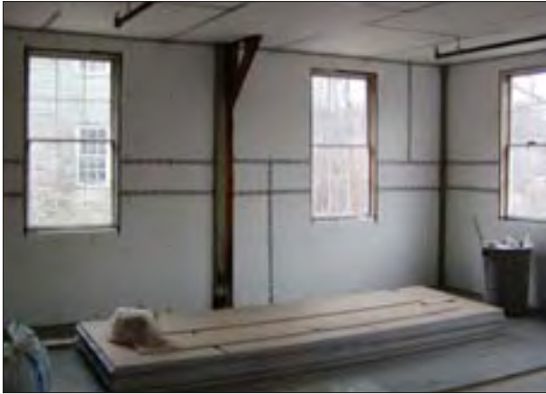
EA45 Interior Rigid Insulation (taped seams for air seal) on Walls
