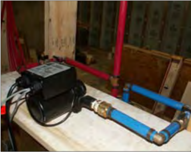
EA78 On-Demand Recirculation Pump for Hot Water
