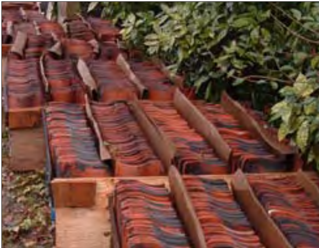
MR108 Salvaged Roofing Tiles Ready for Reinstallation
