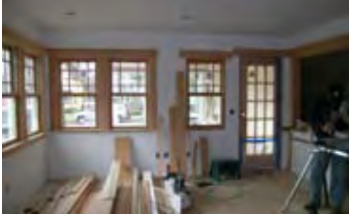
Office during construction
