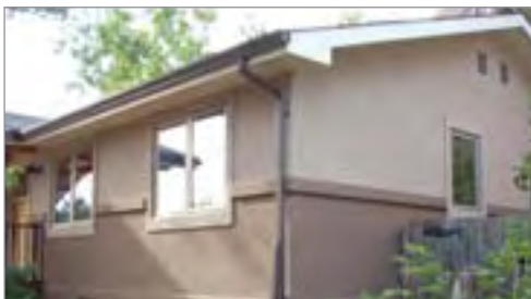
Finished exterior wall
