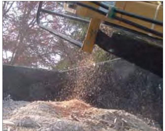
SS39 Clean Wood Waste for Site Erosion Control
