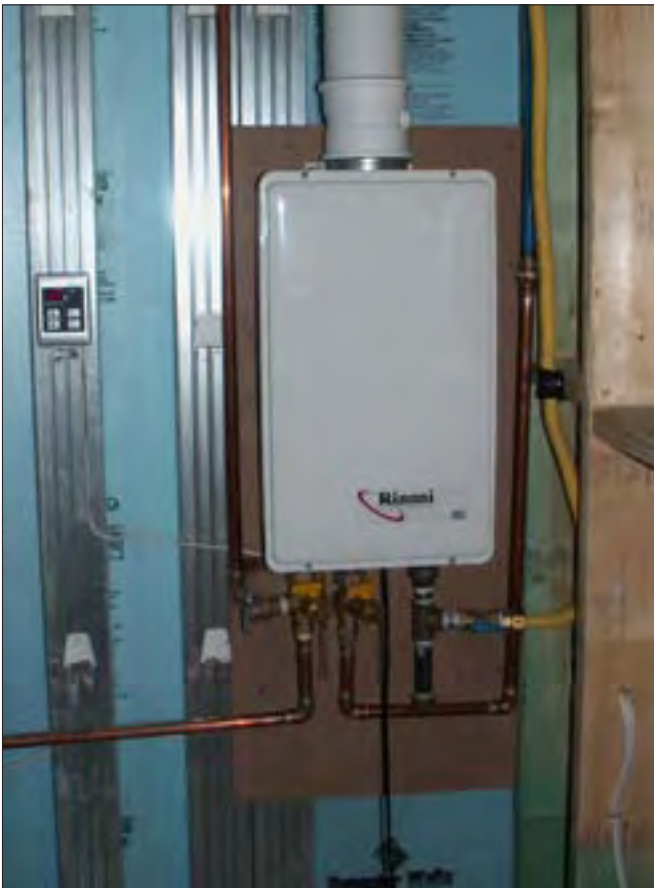
EA79 One Approach to Efficient Water Heater: Gas Tankless
