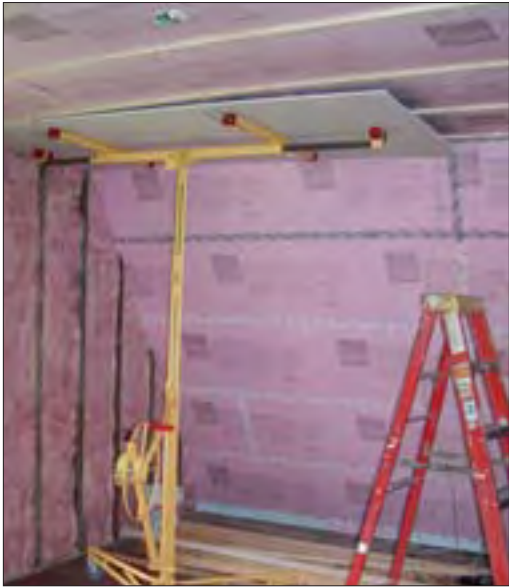
EA45 Interior Rigid Insulation and Air Sealed (taped seams) on Ceiling
