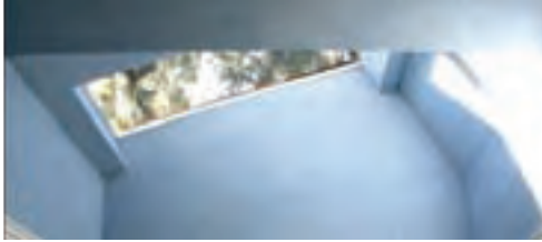
Skylight in shower stall
