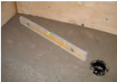
Durable shower pan – under construction
