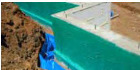
Water-managed, ICF crawlspace foundation
